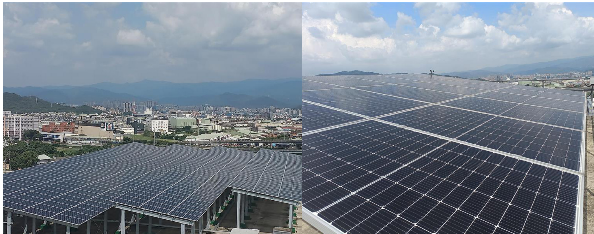
⑦ Rooftop Solar Power System at the Bade Plant
